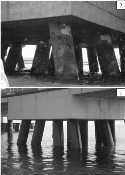
图 5 码头修复前后外观：(a)施工前，(b)施工后 Fig. 5 The appearance of the pier before and after repairing with PTC
